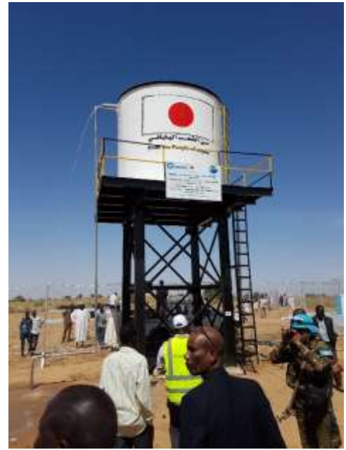
Water Yard constructed in Tanjiki
